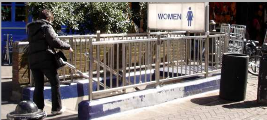
Figure 3: Carnaby Street Public Toilets 30
